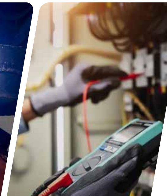
ELECTRICAL/ELECTRONIC CONTROLS TECHNOLOGY
