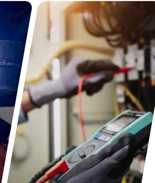
ELECTRICAL/ELECTRONIC CONTROLS TECHNOLOGY
